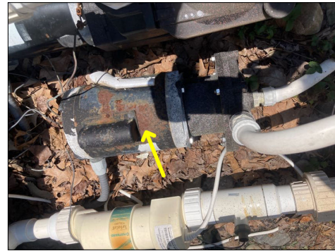
Rust and corrosion - booster pump
