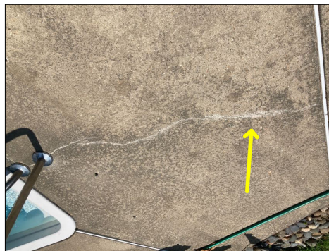
Deck cracking
